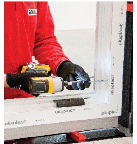
14 Fix the windows mechanically
