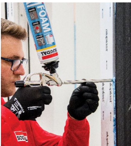
15 Remove spring clips and seal connection joint between frame and window
