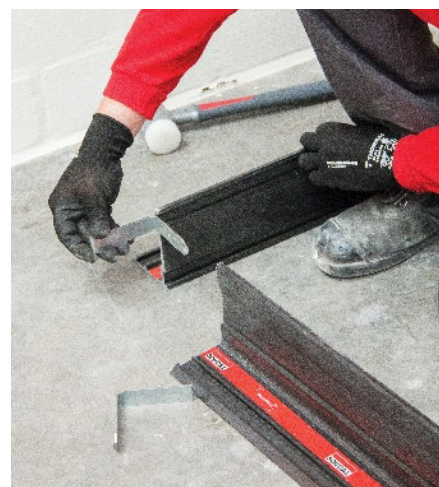
03 Insert the corner connector
