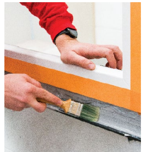
17 Seal with Soudatight Hybrid on the outside
