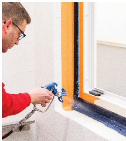
16 Seal on the inside with Soudatight LQ / SP
