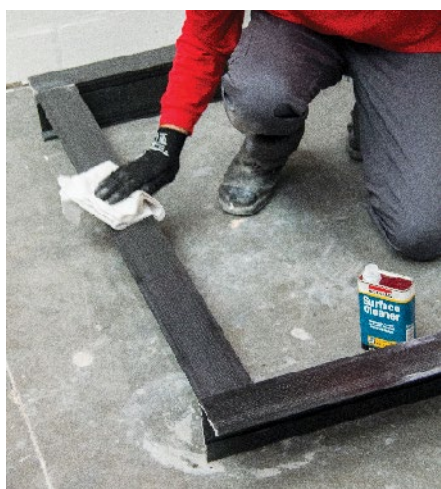
06 Clean the backend of the frame
